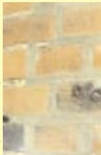
Inappropriate and unnecessary repointing carried out in cement. The original penmanship pointing is shown to the left
