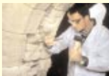
A skilled mason using specialised tools to clean a stone joint
