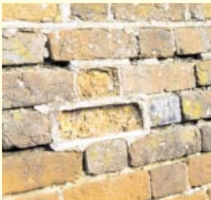
Repointing with an inappropriate hard cement mortar has caused the bricks themselves to decay
