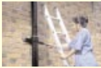
Repainting a cast-iron downpipe
