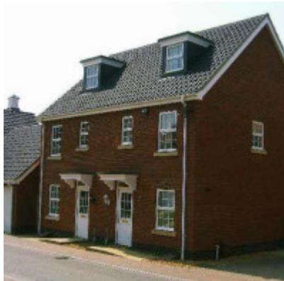
A new 4-bed semi-detached house built by Persimmon Homes in a new development of similar houses built in 2006. It is a timber-framed construction with a brick façade built to 2002 Building Regulations standards.
